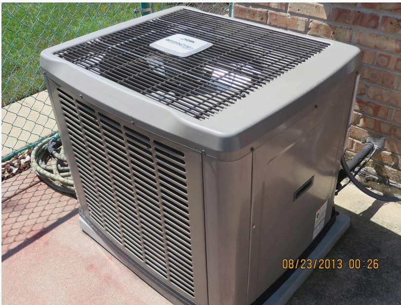
Photo 1: Rear yard, west side of house
